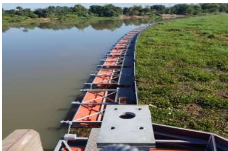
Figure 4: Aquatic weeds with a dominance of Water Hyacinth trapped by a weed boom recently installed upstream of Kamuzu Barrage on the Shire River in Malawi (Source: Peaches Phiri, 2019)
